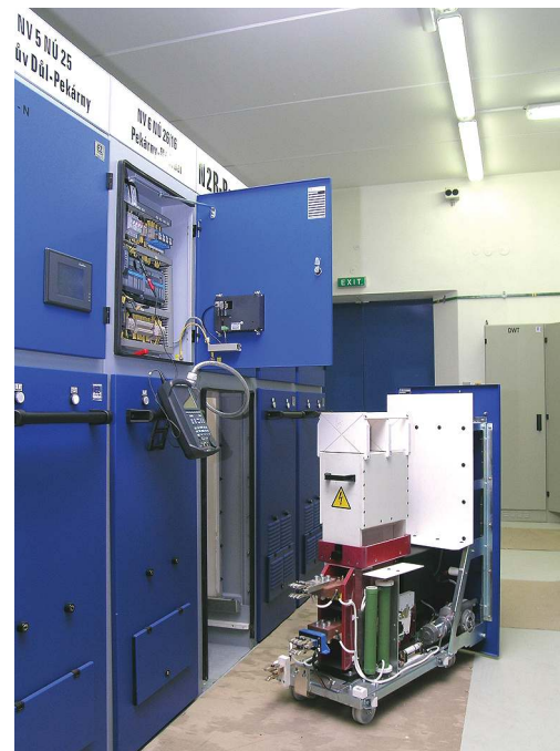
Section of the withdrawable high-speed circuit breaker
